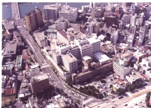
Before the removal of former main building [April, 1992]
