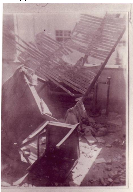
North hospital ward 2nd floor nurse office
